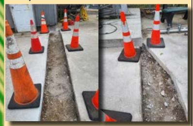
Now all we have to do is the digging, we will need help with that step, and with laying in the pipe for the feed lines and control cables to the tower – and then to the building. We will also be installing a weatherproof electrical box where the feed lines and control cables will be terminated.
